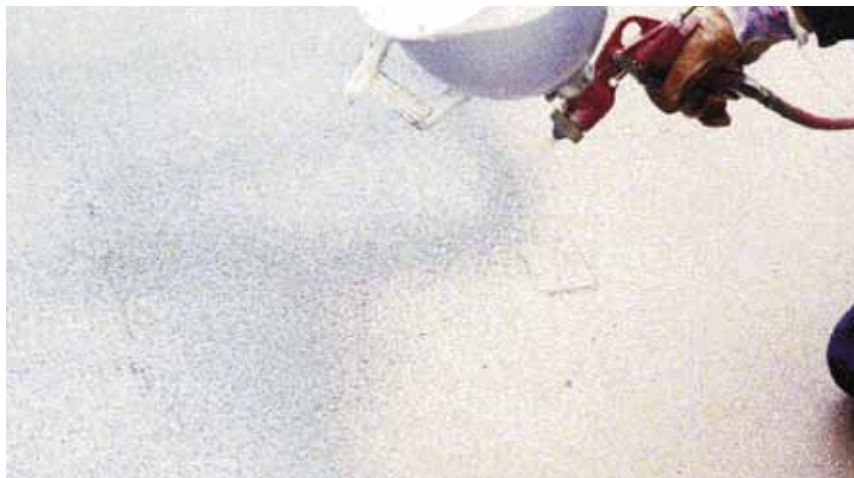
8. Application – circular motion should be used
