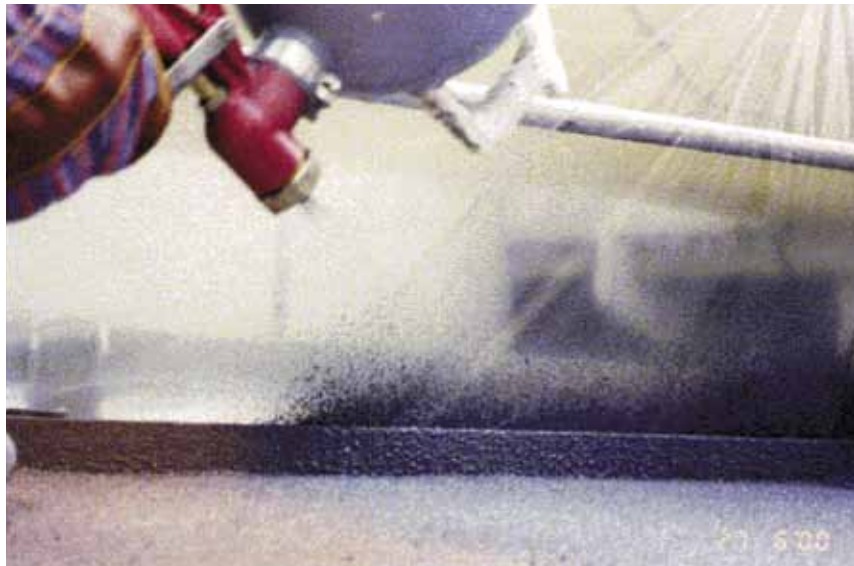
7. Application – circular motion should be used
