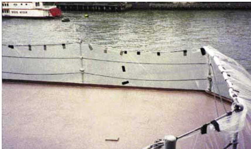
5. Pre-primed deck with Jotamastic masked off because of overspray
